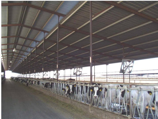
Figure 4-4. Example of circulator fans mounted over cows’ backs over the feed alley
