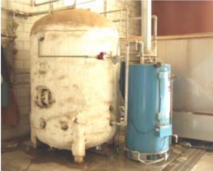
Figure 5-4. Conventional water heater with storage
