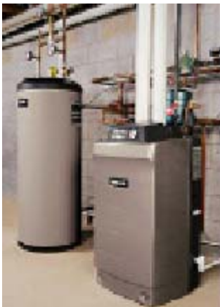
Figure 5-6 High efficiency water heaters.
