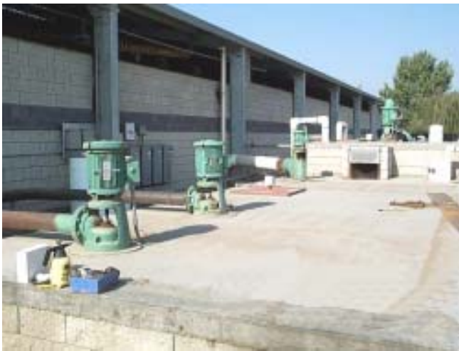
Figure 6-6. Intermediate water storage reservoir on California dairy
