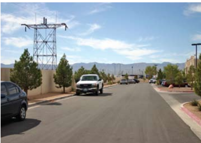
Existing view of 115 kilovolt transmission line facing west from Primm Valley Casino Resorts in Primm, Nevada.
