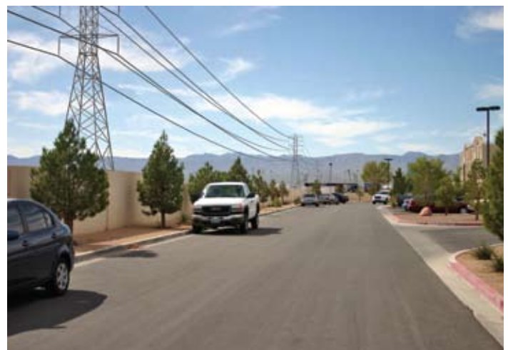
Simulation of proposed 220 kilovolt lattice steel structure transmission line facing west from Primm Valley Casino Resorts in Primm, Nevada
