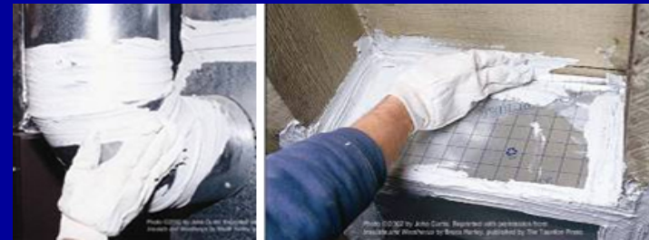
Application of mastic
